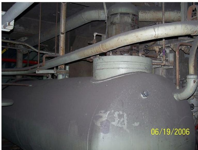
*Figure 5: Liquid Mercury Storage Tank.*
