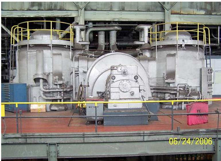
*Figure 1: Mercury Turbine-Generator (center) and Mercury Condenser (either side).*
