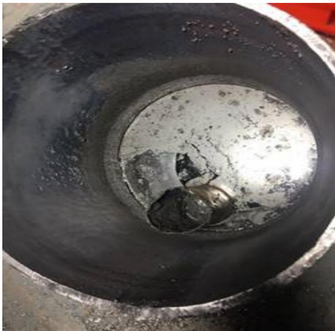
***Figure 13: Liquid mercury found in equipment***
